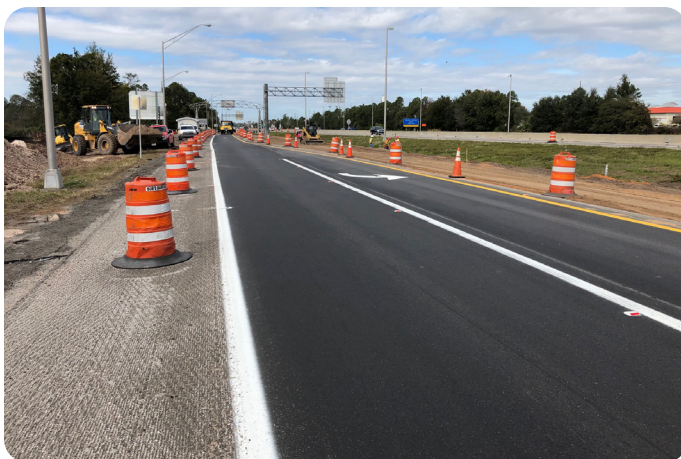
Pavement markings keep motorists aware of lane shifts
