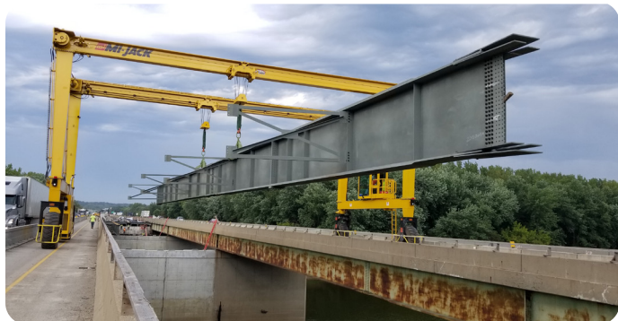
Innovative beam erection techniques to minimize traffic impacts and increase safety on the INDOT I-65 over the Wabash River project.
