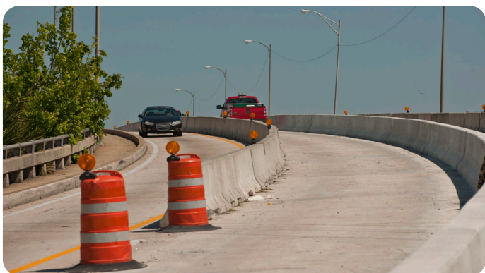
Temporary traffic barriers increase safety for both crews and the traveling public
