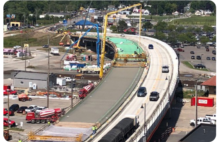
Superior Construction safely building adjacent travelers on the INDOT US 35 Bridge Replacement project.
