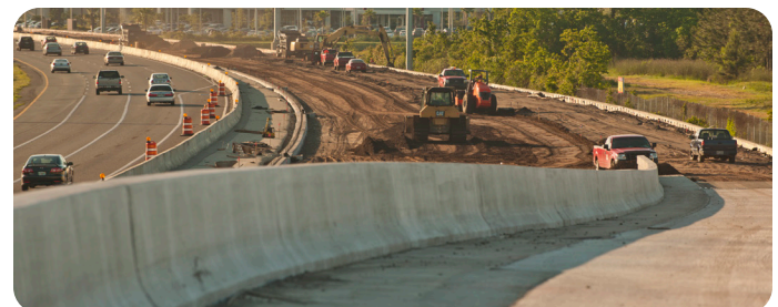
Interchange construction with limited movement closure durations.
