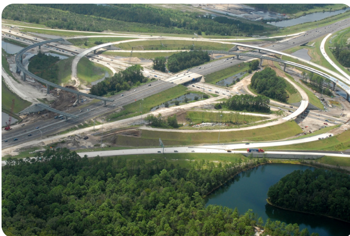
Superior Construction building system-to-system interchange in busy urban area.
